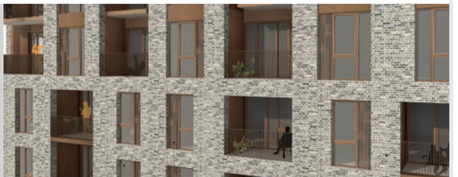
FEATURE REAR BUILDING – BLOCK 2 DETAIL
